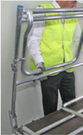
Rotate top section of guardrail through 180 degrees to allow both sections of guardrail to be locked together (at Guardrail locking device).
