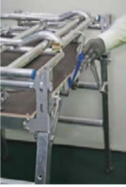
Attach the retaining straps.
