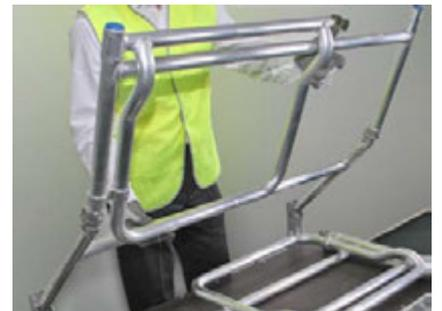
Undo retaining straps and lift one side guardrail section.
