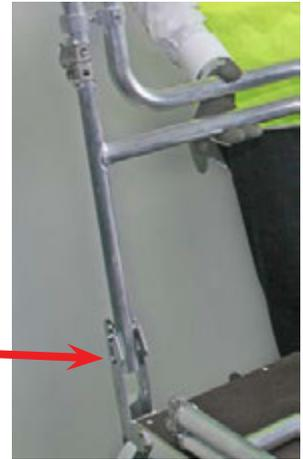
Double check that locking positions at base of the guardrail are firmly secured.
